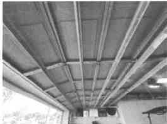
Garage Overhead Door(s): Wind rated or better No decal nor other information evident on overhead door/other for impact rating verification.
